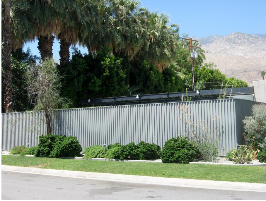
Photo 3: East elevation showing 1992 pool terrace wall replicating original aluminum siding seen elsewhere on the facade. (Author Photo. June 2020)
