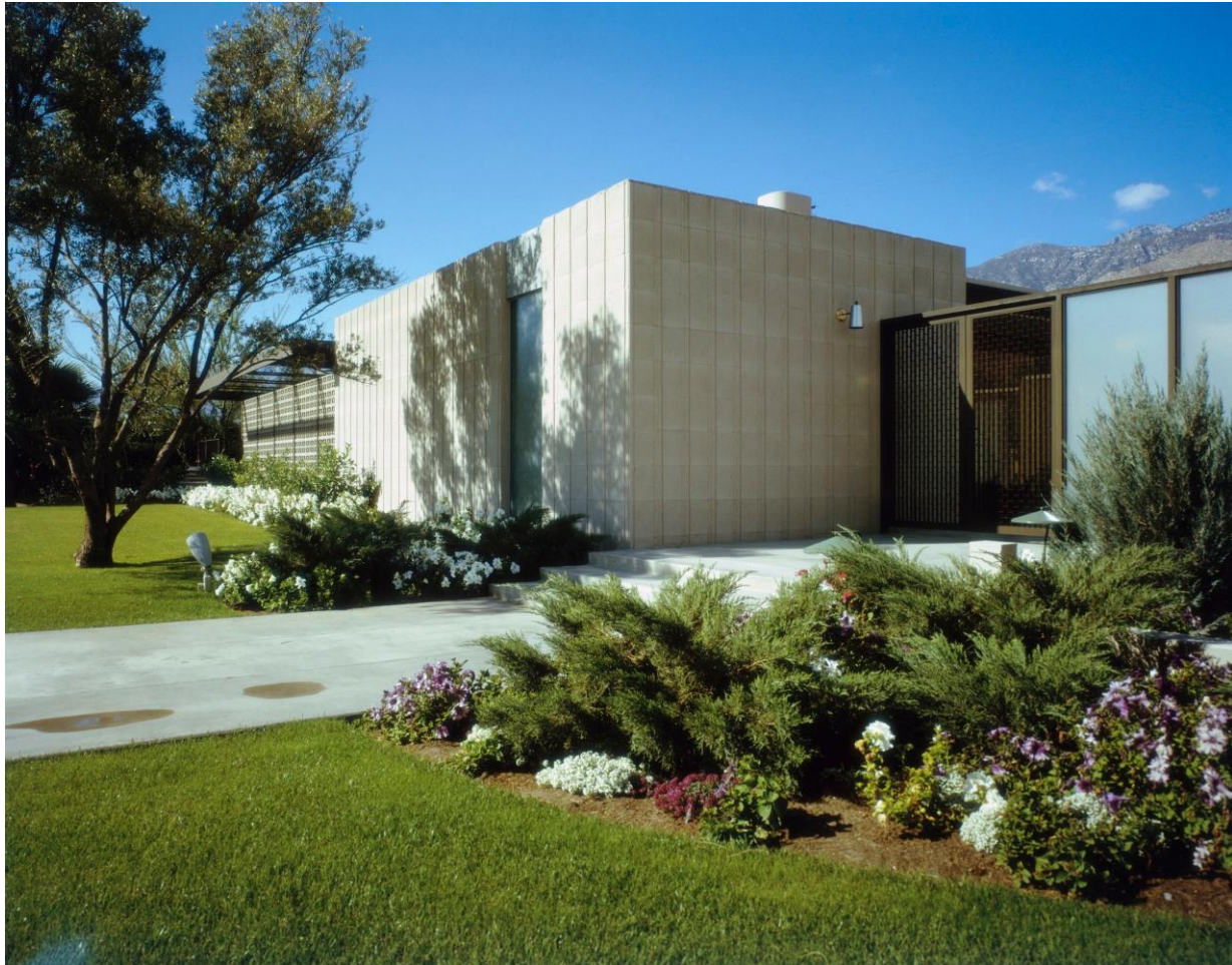
A 1961 Julius Shulman view of the Sutter Residence east elevation showing the variety of exterior materials used - concrete, steel, glass and aluminum. (J. Paul Getty Trust. Getty Research Institute, Los Angeles (2004 R.10))
