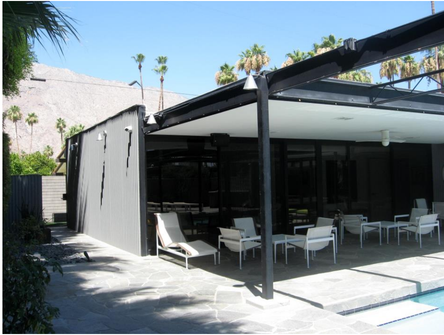
Photo 11: View looking west showing terrace in front of master bedroom. (Author Photo. June 2020)
