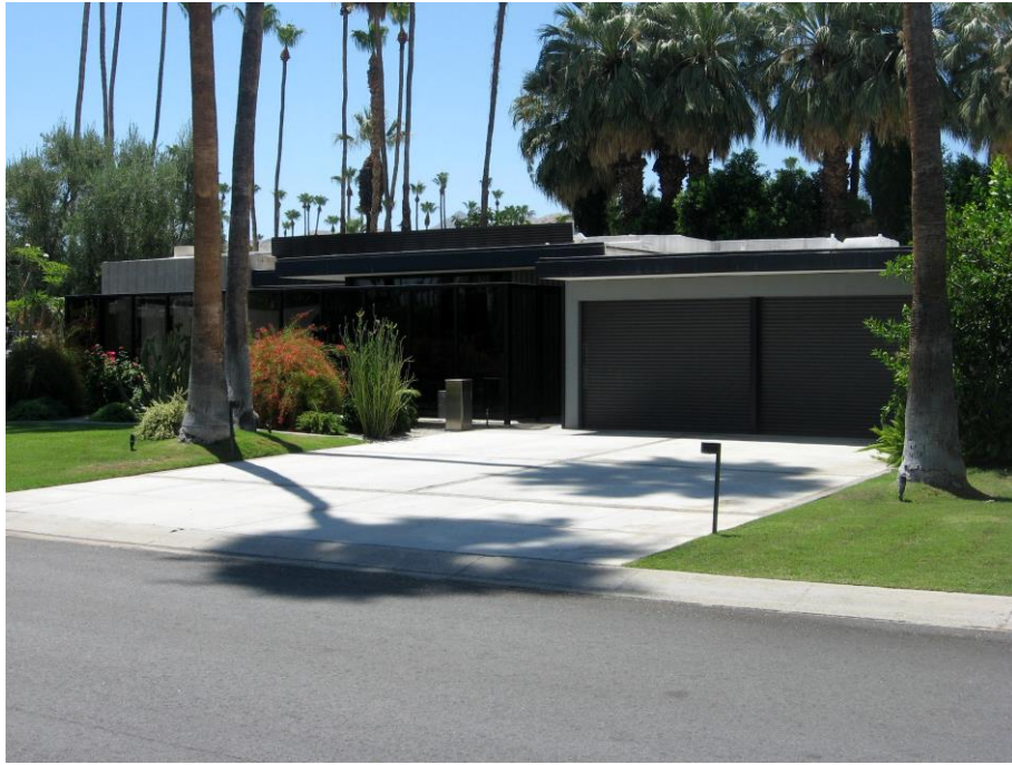
Photo 15: North elevation showing garage and glassed-in entrance patio. (Author Photo. June 2020)
