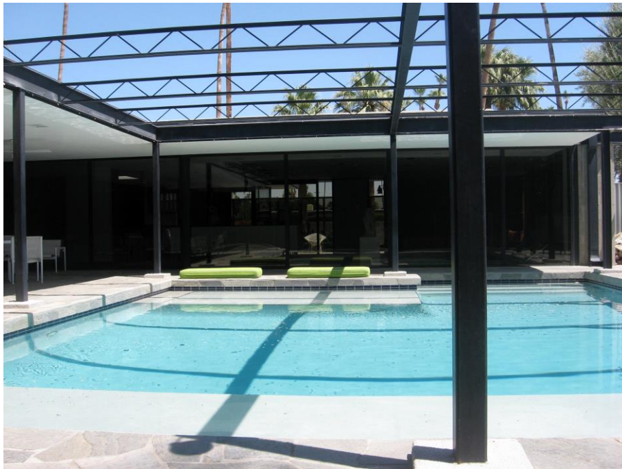
Photo 5: View to west across pool terrace showing original girder trellis. (Author Photo. June 2020)
