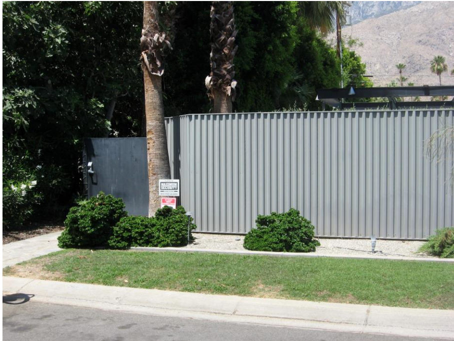
Photo 4: East elevation. Showing aluminum wall and gate to pool. (Author Photo. June 2020)
