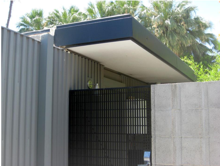
Photo 14: Juncture of west and north elevations showing service yard. Note aluminum siding and concrete block walls. (Author Photo. June 2020)
