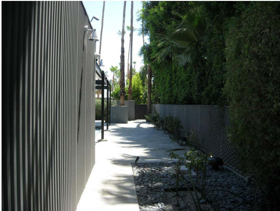
Photo 12: Looking east with south elevation on left. Note original aluminum siding wall. (Author Photo. June 2020)
