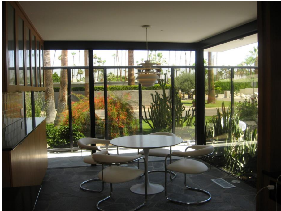
Photo 20: Breakfast room addition was created by extending the house out over a former planting bed. Steel framed windows match original. (Author Photo. June 2020)
