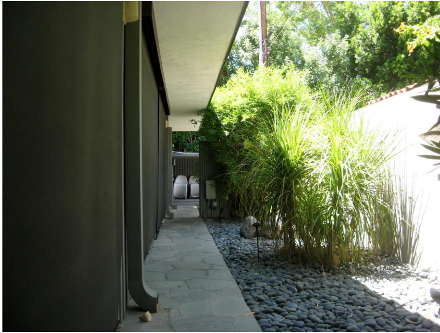
Photo 13: Looking south with the home's west elevation on the left. Windows are shaded by sun screens. (Author Photo. June 2020)
